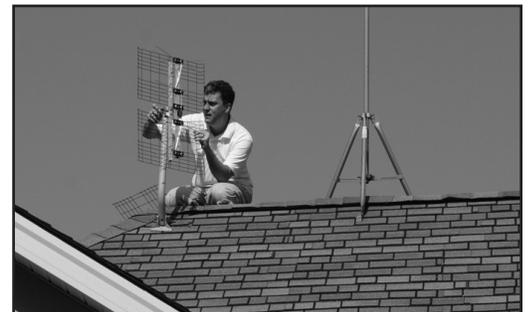
If your signal is weak, check the length of your cable run (the shorter the better) and remove any splitters or diplexers. Check all connectors/junctions for secure fit or corrosion. If your cable run must be longer than 75 feet, or you must use a splitter, consider a pre-amplifier-- [http://www.antennasdirect.com/antenna\\_amplifier.html](http://www.antennasdirect.com/antenna_amplifier.html).
